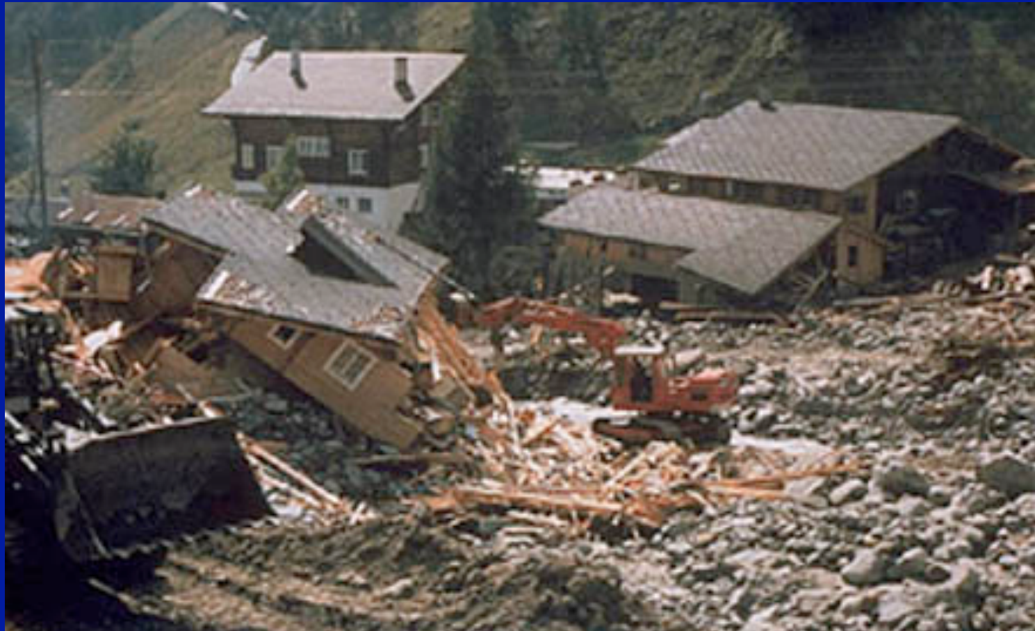
Houses undermined by melting Permafrost
